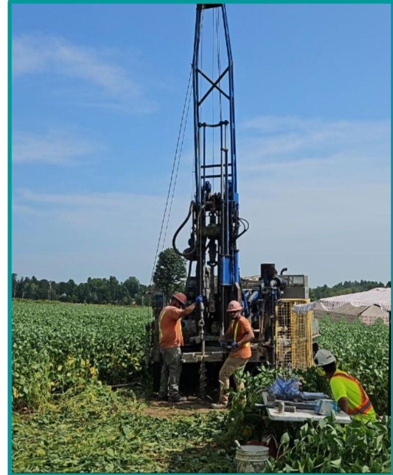
Borehole Investigations and Monitoring Well Installation (AECOM, 2025)
