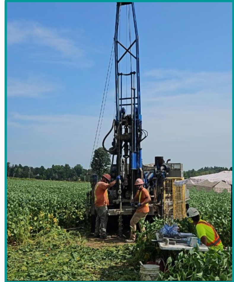
Borehole Investigations and Monitoring Well Installation (AECOM, 2025)
