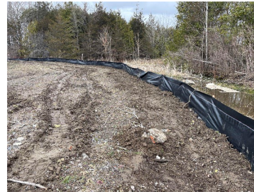
Erosion and Sediment Control Fence Protection of Adjacent Watercourse
