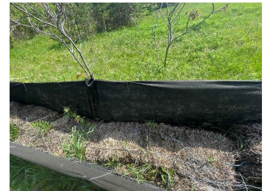
Erosion and Sediment Control Fence delineating the Work Area
