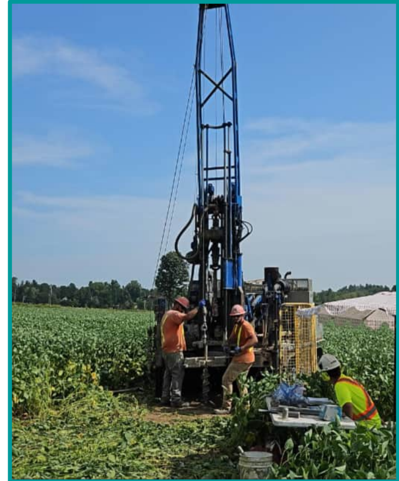
Borehole Investigations and Monitoring Well Installation (AECOM, 2025)
